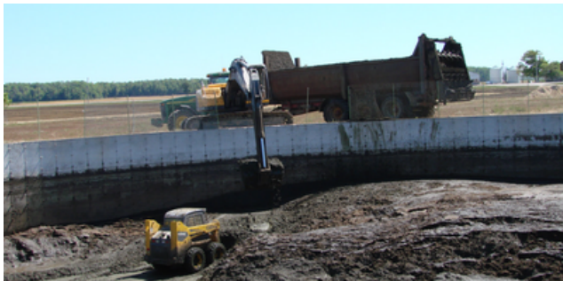
Cleaning out sand-laden manure from a manure pit
